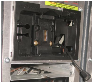
Fig. 7-19 Garmin GPS AERA Power/Data and XM Antenna cables
